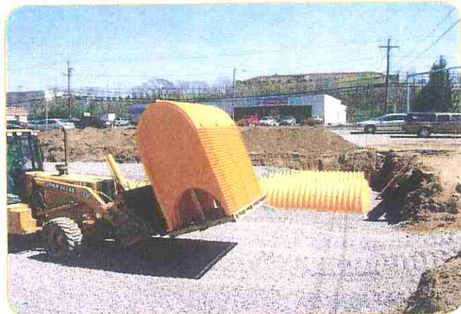
StormTech chambers fit the site's limited zone.
